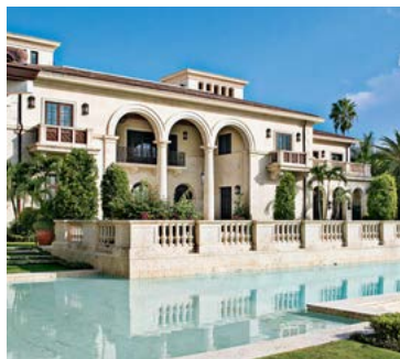
EXTERIOR FINISHING & RESTORATION
