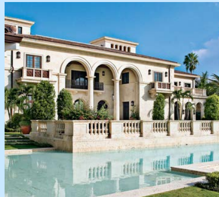
EXTERIOR FINISHING & RESTORATION
